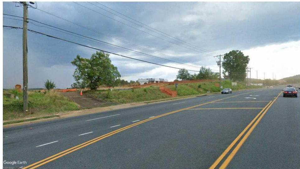
1. ENTRANCE LOOKING NE
