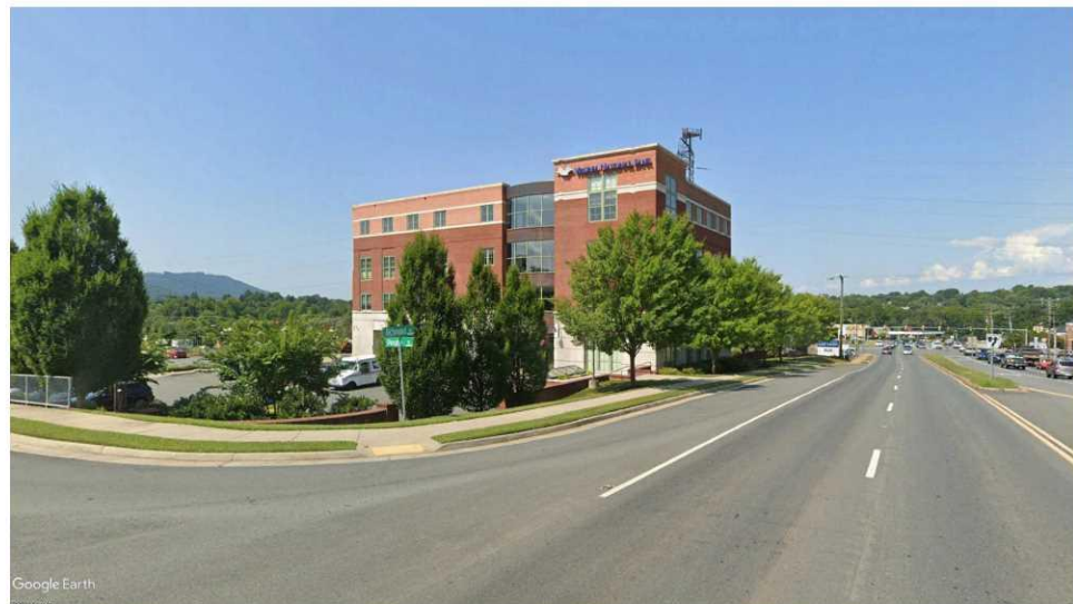
7. EXISTING VIRGINIA NATIONAL BANK
