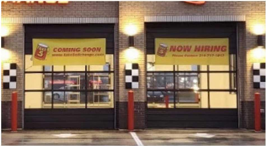
METAL ROLL UP GARAGE DOORS WITH GLAZING
